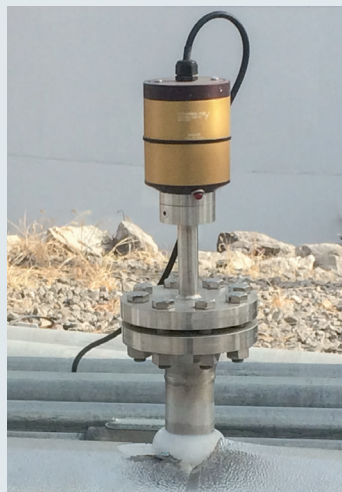
Pilot LNG probe installed at an LNG truck loading facility.
